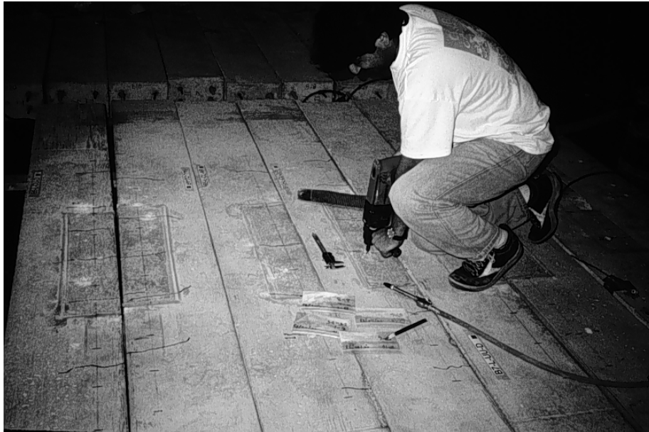
Figure A.57 Sampling chloride from beams before autopsy.
