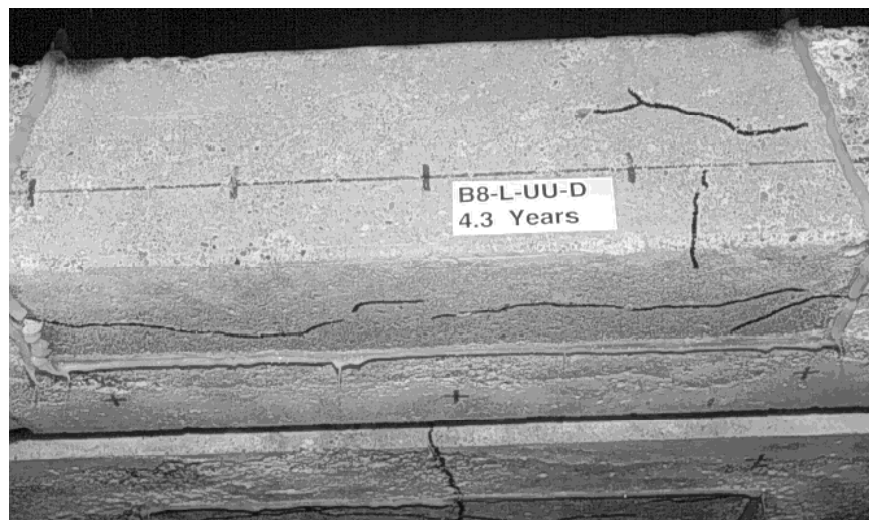
Figure 2.32 Cracking on non-precracked beam B8.
