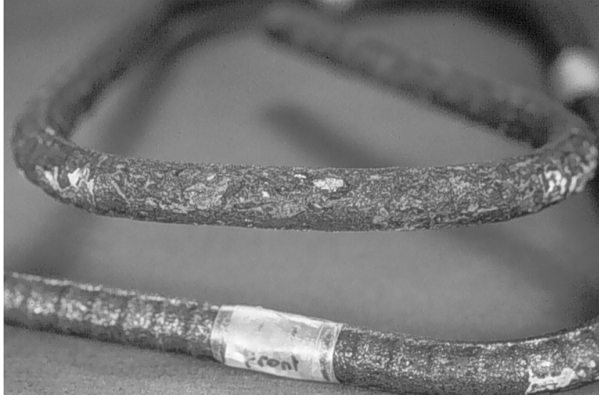
Figure 3.24 Stirrup leg near the beam front surface (top in photo) is corroded while stirrup hook is mottled (bottom in photo) (Beam B32).
