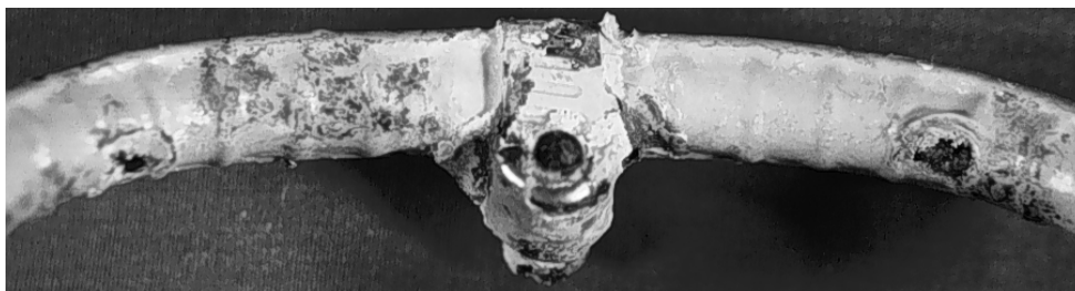
Figure 2.53 Corrosion at areas of contact between stirrup and uncoated bars at one year.
