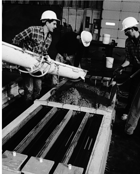
Figure A.13 Casting beam specimens.
