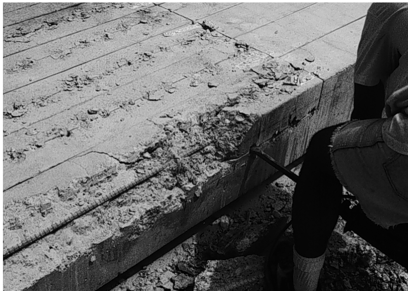
Figure A.59 Beam demolition for bar retrieval.
