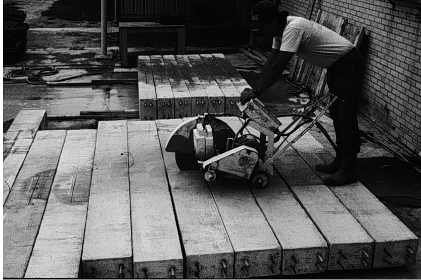
Figure A.58 Saw used to crosscut beams.
